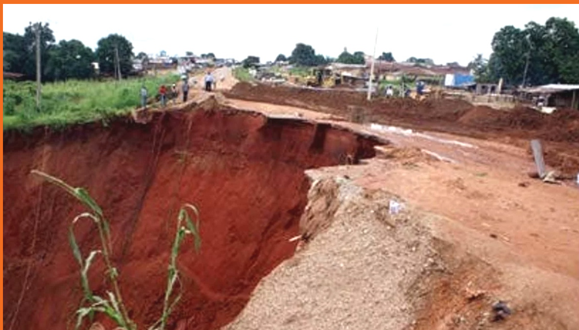
Figure 1: Gully erosion severs road to Owerri [Source: DailyPost]
